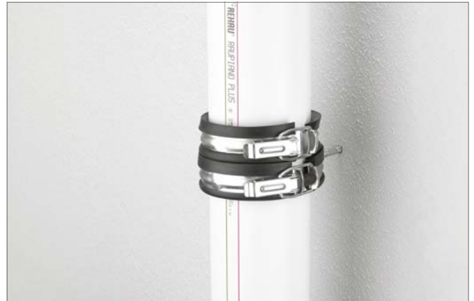
Fig. 7-3 Fully installed support bracket
