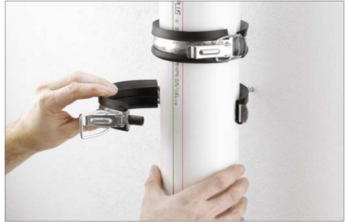
Fig. 7-2 Closing supporting clamp
