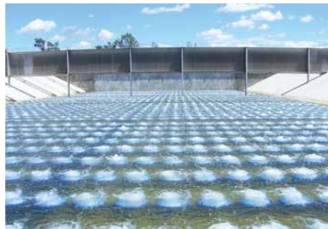
Installation of RAUBIOXON disc aerators at Tamworth WWTP (Australia), 2011
