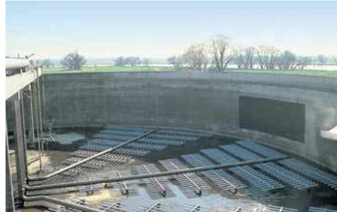
Refurbishment with RAUBIOXON pipe aerators at Wittenberg STP (Germany), 1998
